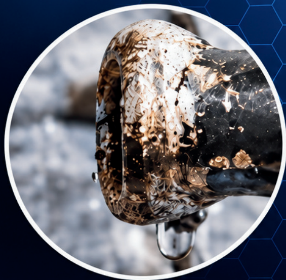
SHORTER LIFESPAN FOR APPLIANCES AND PLUMBING
